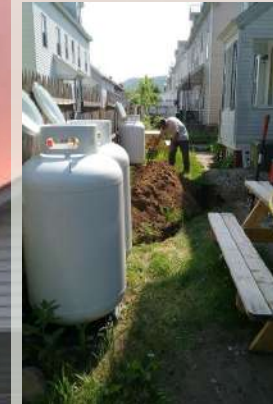
120 Gallon Tank Being Installed
