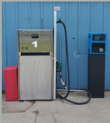
New Diesel Fuel Pump Installed June 1st 2021
