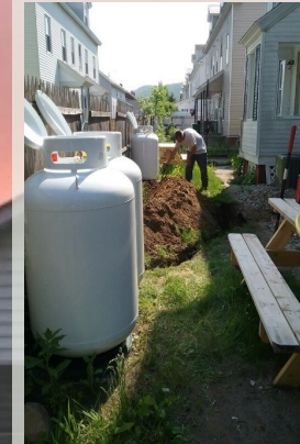
120 Gallon Tank Being Installed
